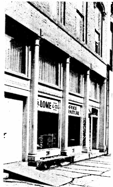
The distinctive features of the Cole Building include cast-iron storefront columns (below) and decorative, terra-cotta window hoods (above).
